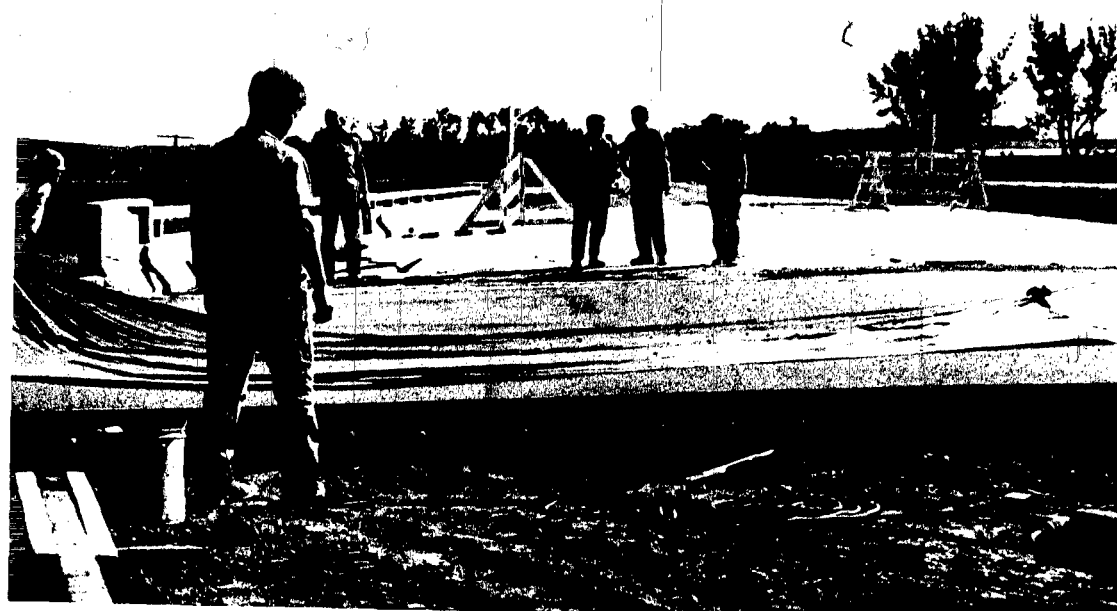
WORKERS TUESDAY were pouring concrete at the north end of the new bridge at the south edge of Wayne, taking advantage of good weather to speed the completion of the Highway 15 improvement project. Project Engineer Dale Poshman.
